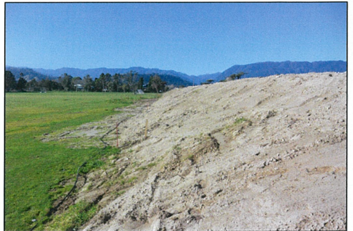
Looking East along final reshaped batters.
