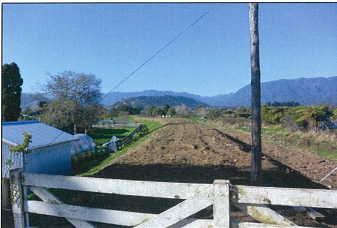
Reformed bank behind Pratts' property looking upstream, showing Anchor pole and wire stay.
